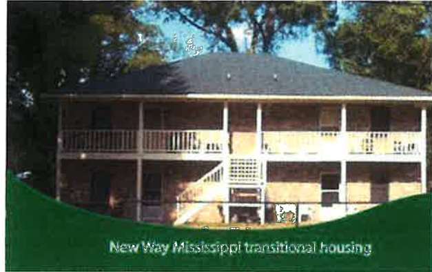
916 Inge St Jackson, MS 39203 Facility Location (26 beds)
